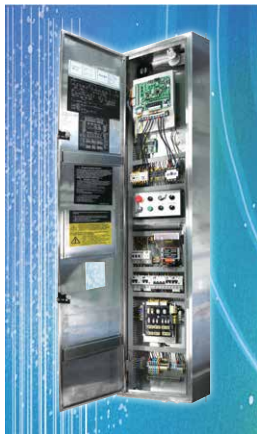
e-com MRL control system
